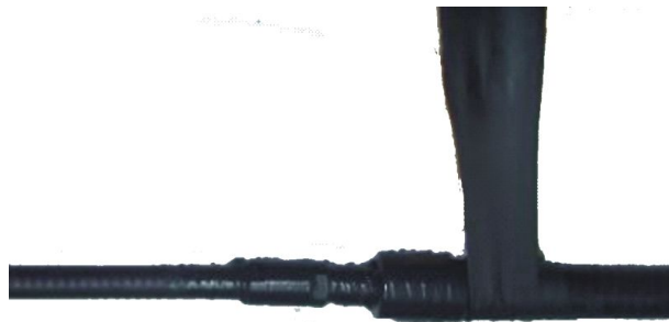
FIGURE 54 WRAPPING THREE LAYERS OF WATER INSULATING TAPE (THE FIRST LAYER)
