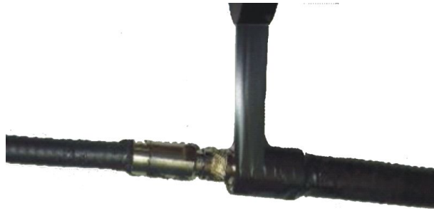
FIGURE 53 WRAPPING A LAYER OF PVC INSULATING TAPE
