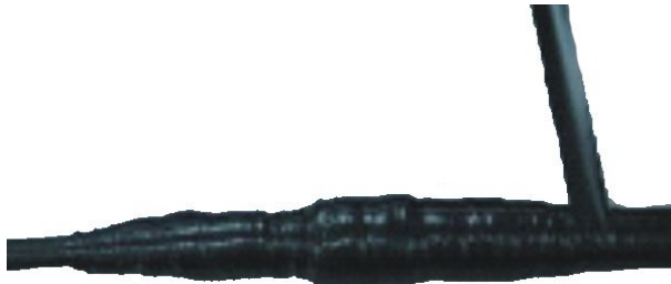
FIGURE 59 WRAPPING THREE LAYERS OF PVC INSULATING TAPE (THE THIRD LAYER)
