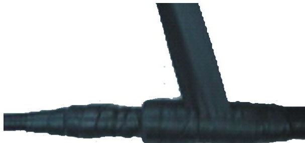
FIGURE 56 WRAPPING THREE LAYERS OF WATER INSULATING TAPE (THE THIRD LAYER)
