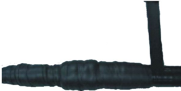
FIGURE 57 WRAPPING THREE LAYERS OF PVC INSULATING TAPE (THE FIRST LAYER)
