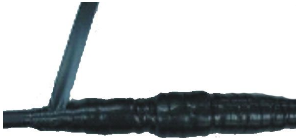
FIGURE 58 WRAPPING THREE LAYERS OF PVC INSULATING TAPE (THE SECOND LAYER)
