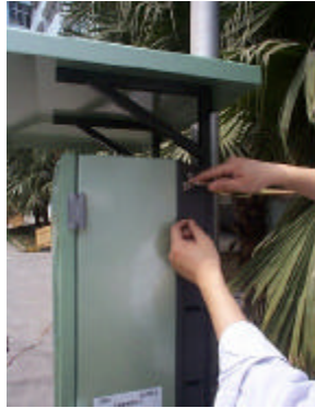
FIGURE 10 FASTENING THE CHASSIS BODY -POLE MOUNTING
