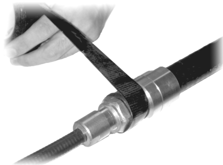
FIGURE 48 WATERPROOF ADHESIVE TAPE WRAPPING (1)
