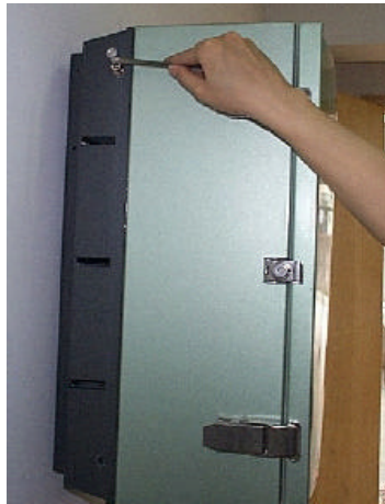
FIGURE 17 FASTENING THE CHASSIS BODY-WALL MOUNTING
