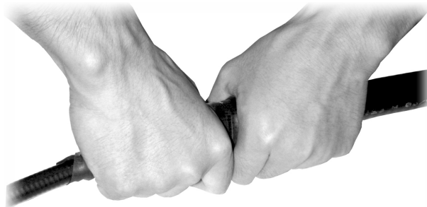
FIGURE 50 WATERPROOF ADHESIVE TAPE WRAPPING (3)
