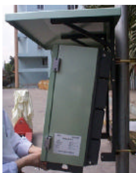
FIGURE 9 PUSHING CHASSIS INTO POSITION-POLE MOUNTING
