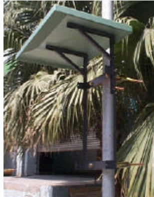
FIGURE 7 SUNSHADE INSTALLED -POLE MOUNTING
