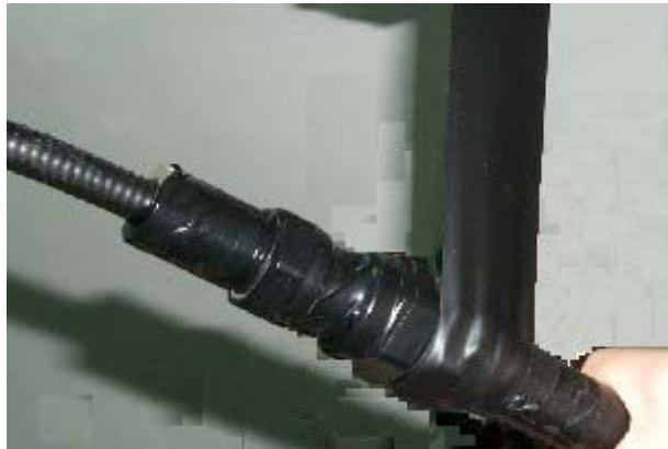
FIGURE 90 WATERPROOF INSULATION ADHESIVE TAPE WRAP
