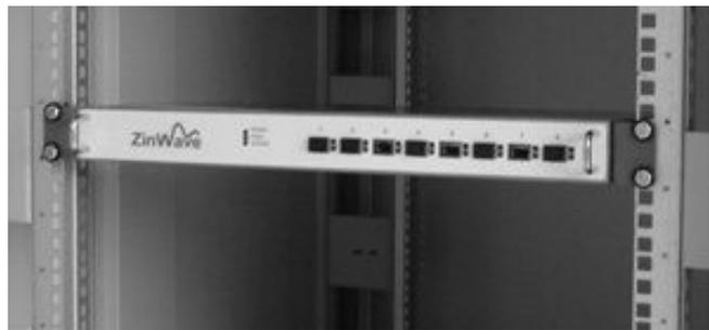
Figure 3-4: Hub Unit mounted into a 19" equipment rack.
