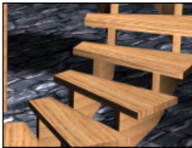
Step depth variance between two stairs
