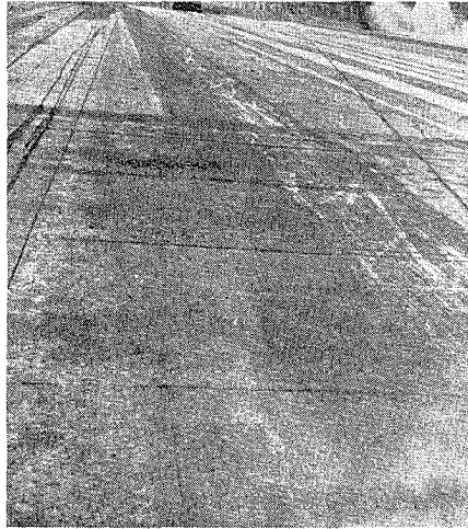
Fig. 4—View looking up spillway face of Grand Coulee Dam showing pitted area at elevation 990 below place where form sprung out of line during construction
