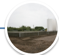
Future Tank space
