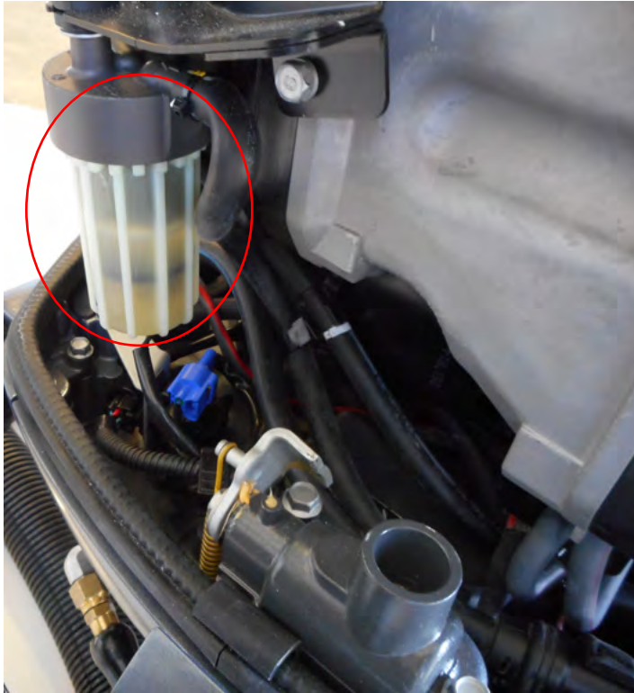
CHECKING ENGINE MOUNTED FUEL FILTER
