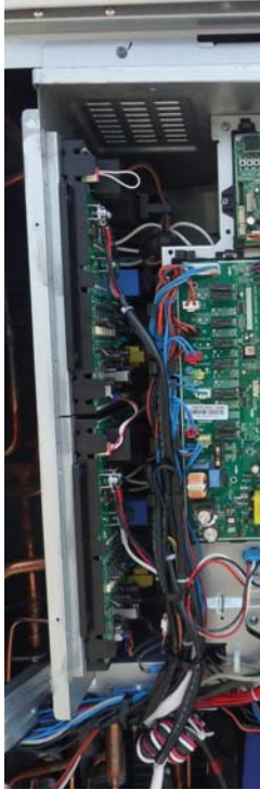
► Comp Wire fix by Holder Wire.
