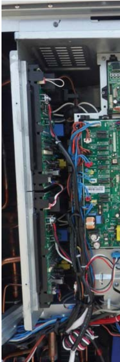
► Comp Wire fix by Holder Wire.
