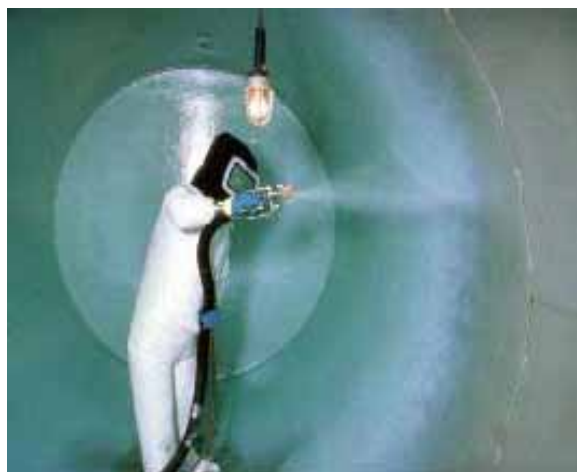
Sample of a Tank being Interior Lined
