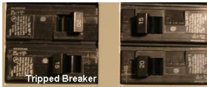
Figure 4 Bottom left corner of picture shows “tripped” breaker.
