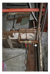
**The building main water shut off** is located in the basement towards O'Farrell. To turn the water off turn red the lever down. Call San Francisco Water district if you are not able to turn the lever.
