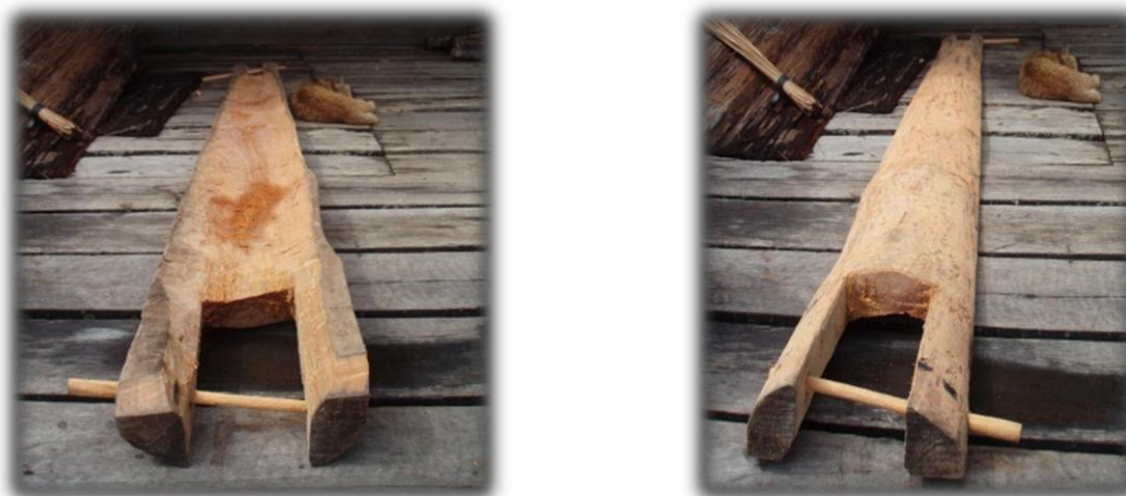
Figure 26: Tikung (rainy season rafters). Photos: Stephen Petersen.
