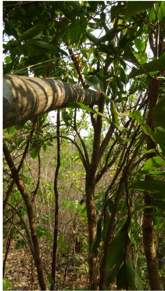
Figure 8: The main rafter beam can be directly mounted between 2 small trees (Mondulkiri, Cambodia). Photos: Eric Guerin.
