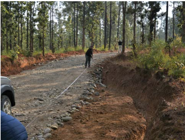
Earthen Side Drain for Water Management
