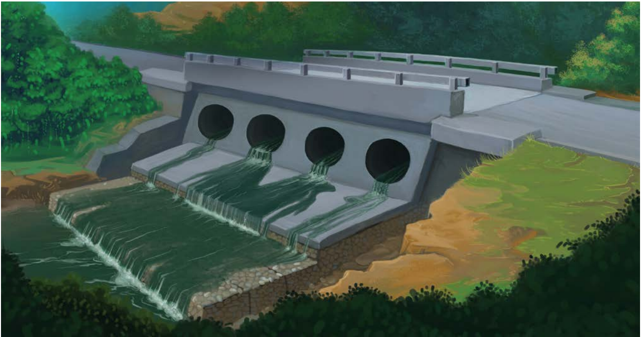
Picture: Outlet of water crossing structure
