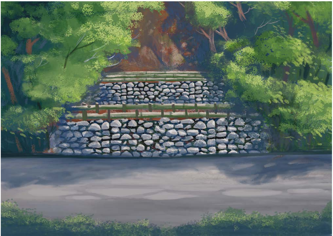
Picture: Low cost earth stabilizing wall
