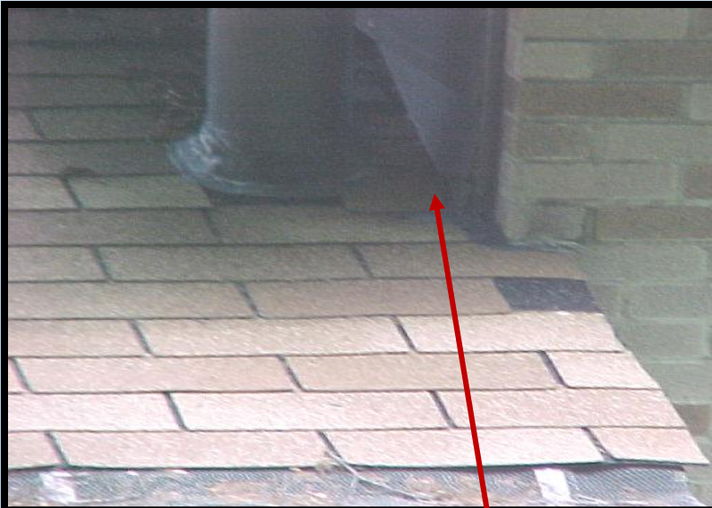
Roof repair at flashing and chimney
