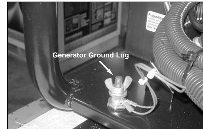
Figure 13 - Grounding the Generator
