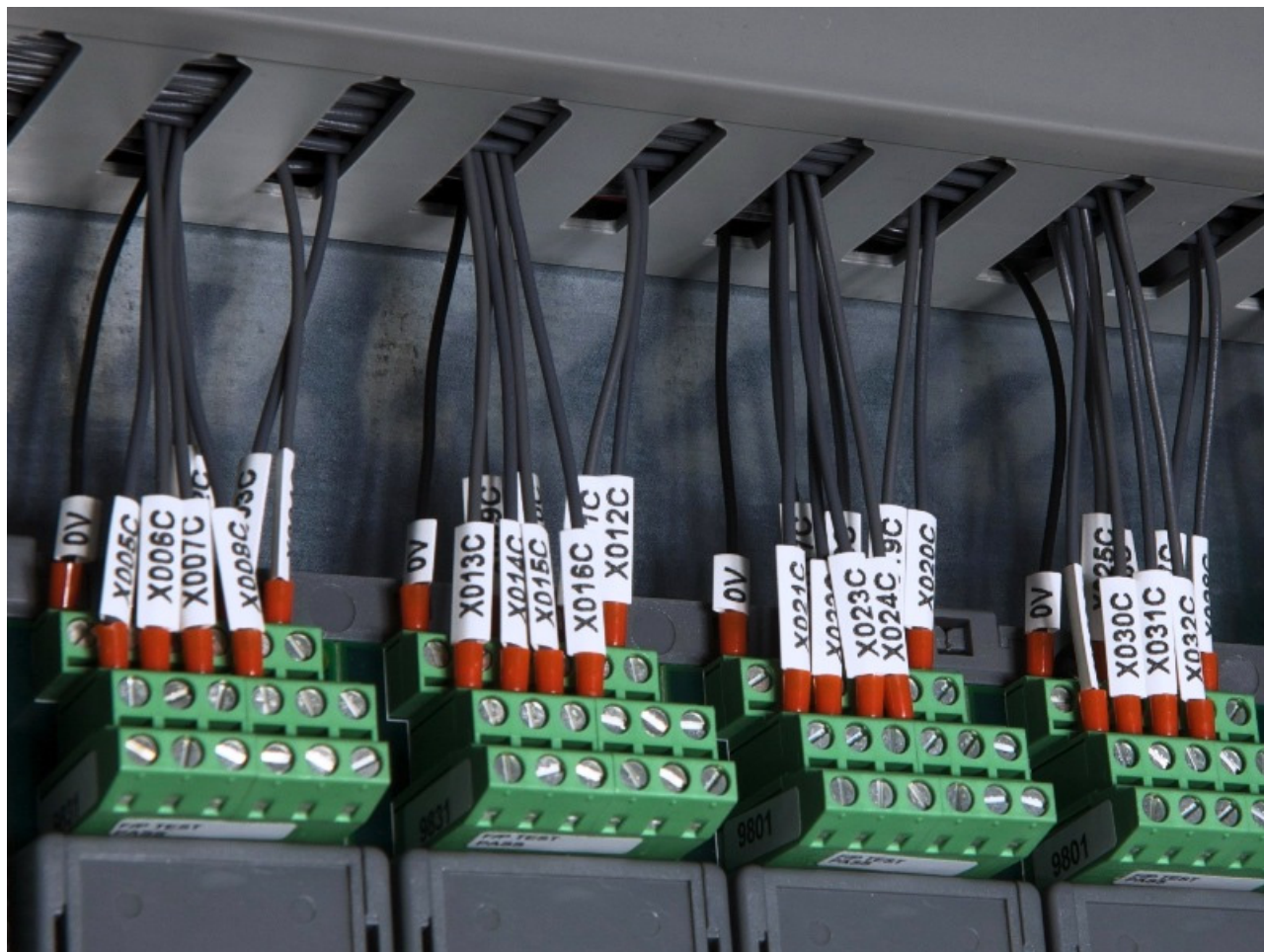
Figure 8 - Field Wiring Connections
