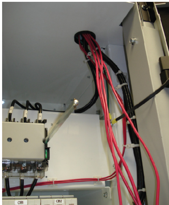
Figure 34 - Route control wires through grommeted cutout
