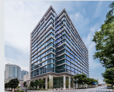
Minatomirai Research Center (Yokohama, Japan)
