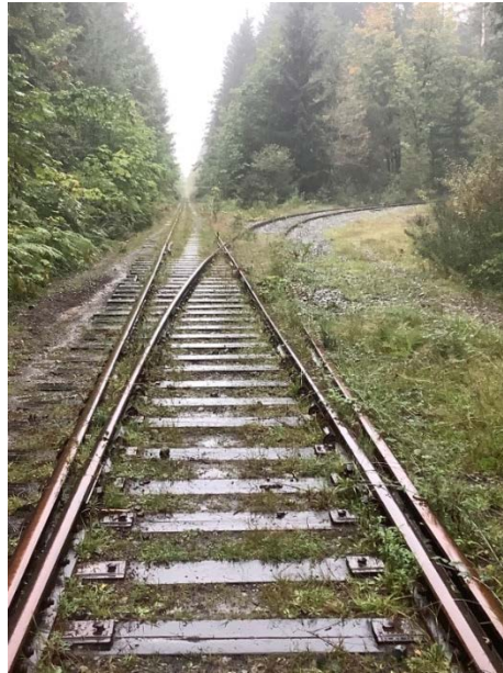
Figure 19: Typical Turnout within Corridor
