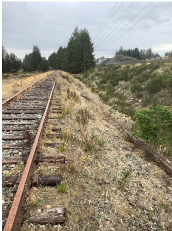
Figure 5: Typical Drainage Ditch Observed at Langford.
