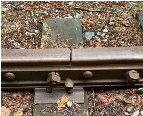
Figure 16: Standard Joint Bar
