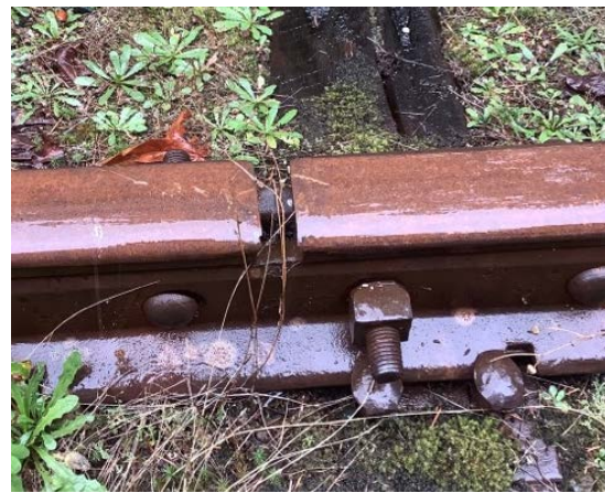
Figure 17: Angle Joint Bar
