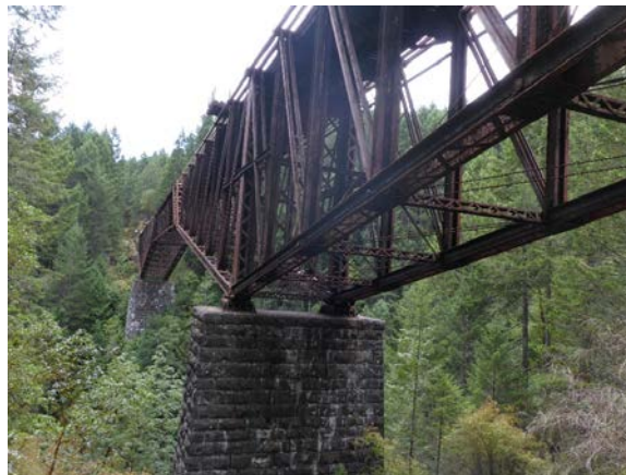
Figure 20: Niagara Canyon Bridge - mile 14.0
