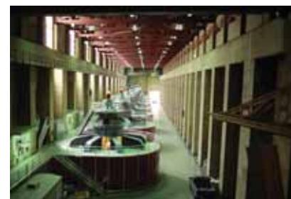
level. Thus when the demand increases, the water may be released back to the lower reservoir, through a turbine. This idea of storing energy is known as pumped storage.
