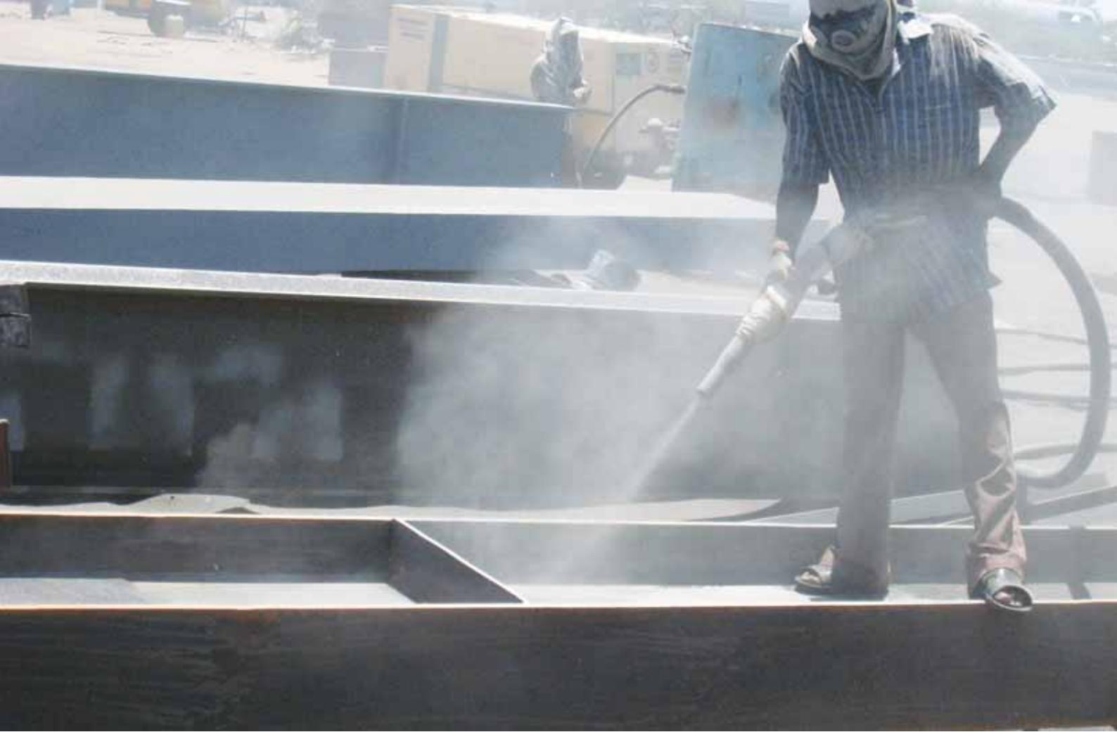
Variants of the abrasive blasting process are known as *bead blasting*, *shot blasting* and *soda blasting*. The abrasive of choice is propelled using a propellant, typically compressed air or pressurized liquid. In the compressed air version, the role of the pressurised air is comparable in importance with that of the abrasive.
