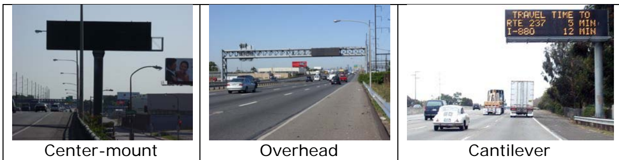
Figure 3-7: DMS Structure Types
