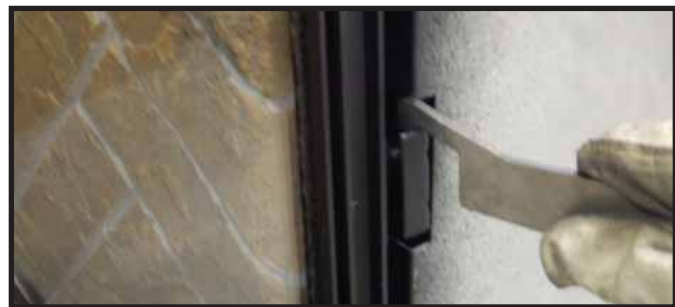
Figure 11.7. Fasten Side Glass Clips
