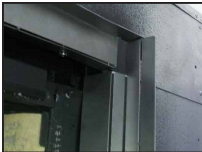
Figure 10.4 Top/Side Finishing Templates Installed
