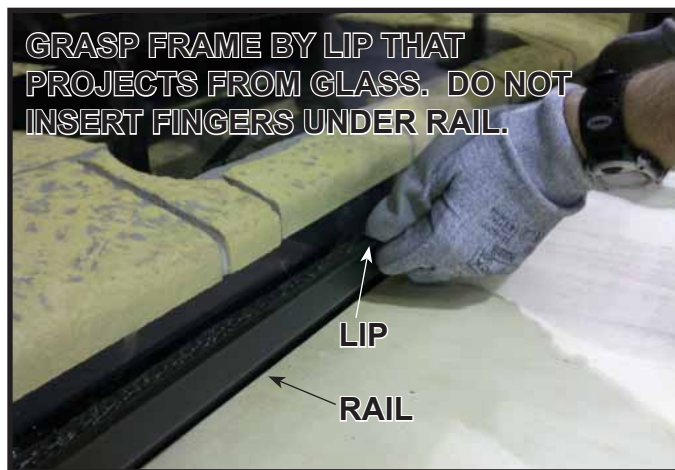
Figure 11.6. Install Glass
