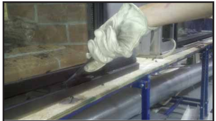
Figure 11.3 Inserting Glass Clip Tool
