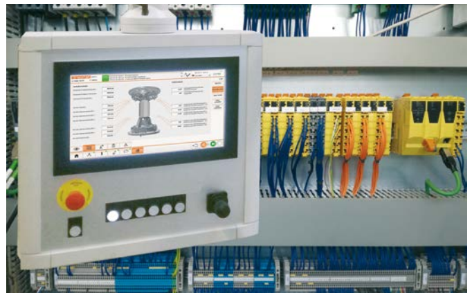
The emergency stop button is linked to the safety controller via an emergency stop console. All the safety components from the electrical plan are implemented in UML.
