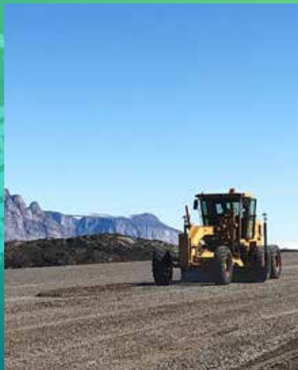
Runway maintenance with machine control in Greenland
