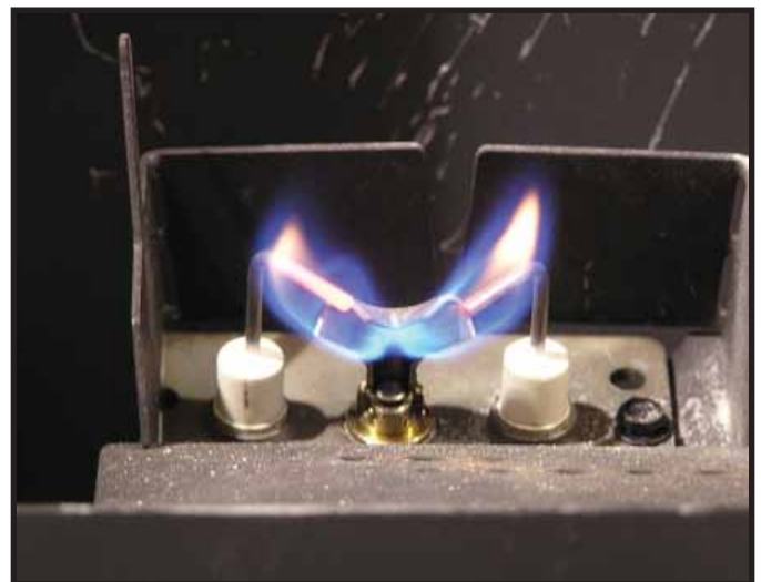
Figure 3.1 IPI Pilot Flame Patterns
