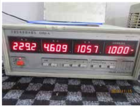
Power check at switch "fan II" and "Heat II"
