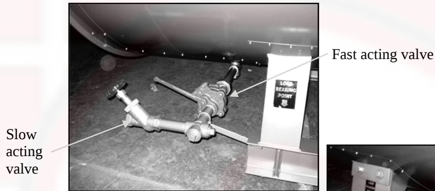
Blowdown valves, single connection: Figure 33
