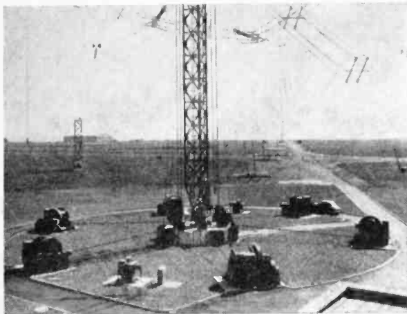
NATO VLF station at Anthorn, England, has six halyard winches around the base of main mast. At the present time it is the largest single antenna system to be found in Western Europe.
