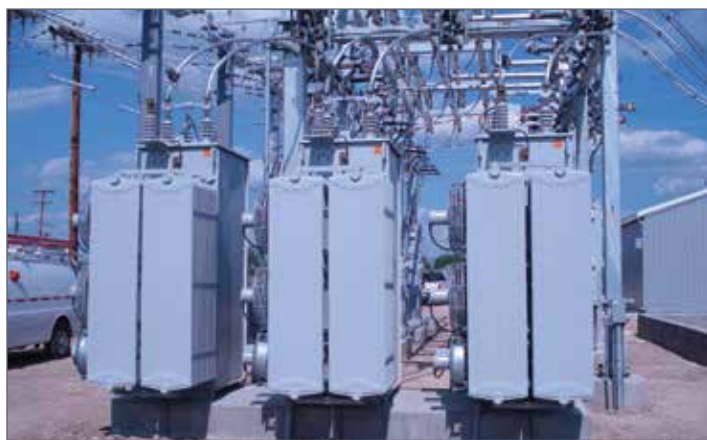
Substation Class Regulators
