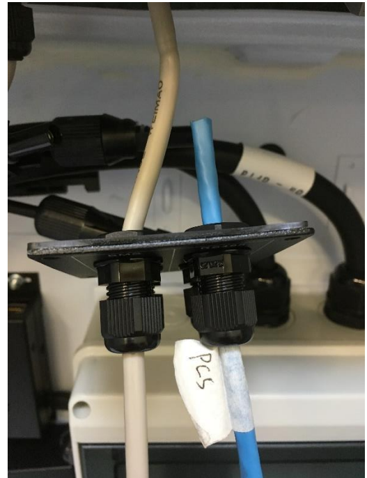
Fig 5: Feed the new PCS cable through the gland
