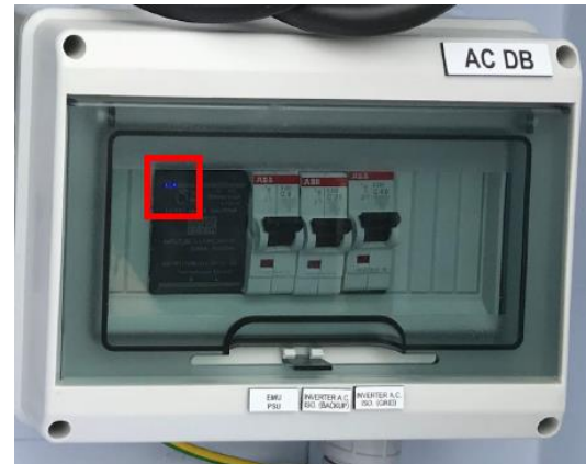
Fig 18: EMU power supply LED
