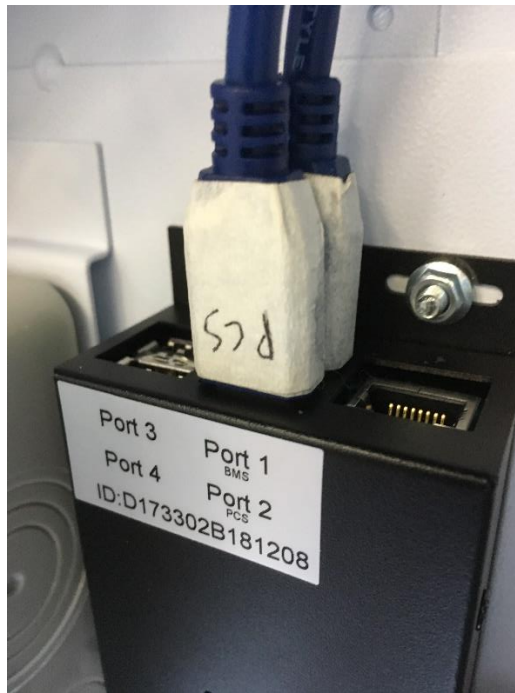
Fig 7: PCS and Battery RS485 connection
