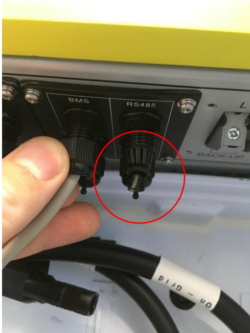
Fig 2: Cut the existing USB cable
