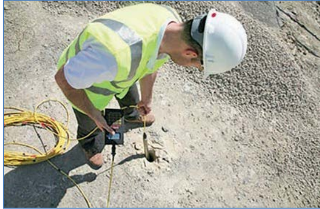
Figure 19 Deploying the probe into the borehole
