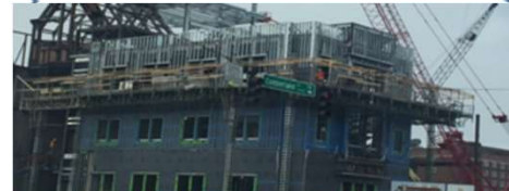
UT Student Union Concrete designed with Kingston Fly Ash
