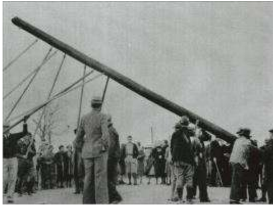
First power pole erected in 1934 in Pontotoc, Miss.
