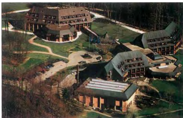
In 1988, the training centre of Haus Lammerbuckel on the Schwabische (Swabian) Alb was extended by the building at top left of the picture. Last year, over 600 training courses were held, with a total of 11,000 participants.
