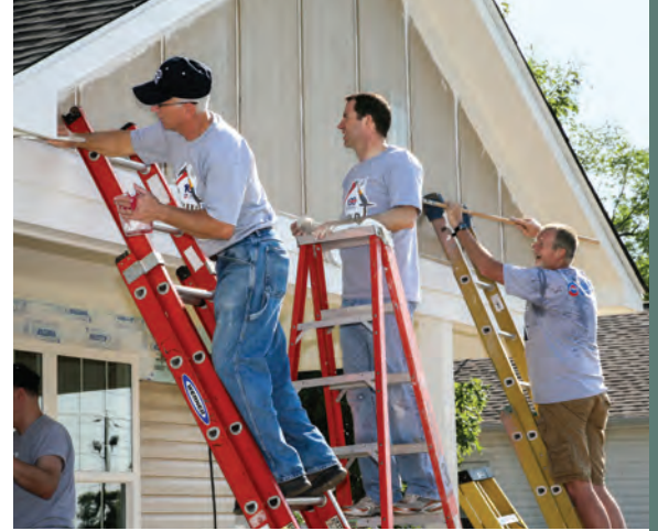
Employee House Build
