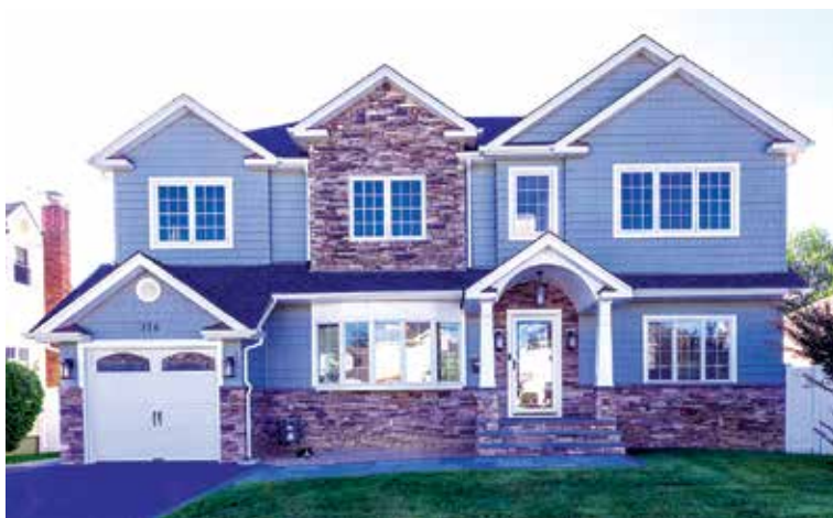
Photo Courtesy of Noah Construction & Builders 2019 Platinum CoTY Winner / Residential Addition over $250,000
