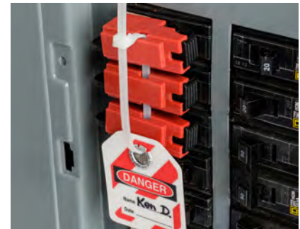
120V breaker lockout devices fit on breakers next to each other, enabling multiple tagouts at one time
