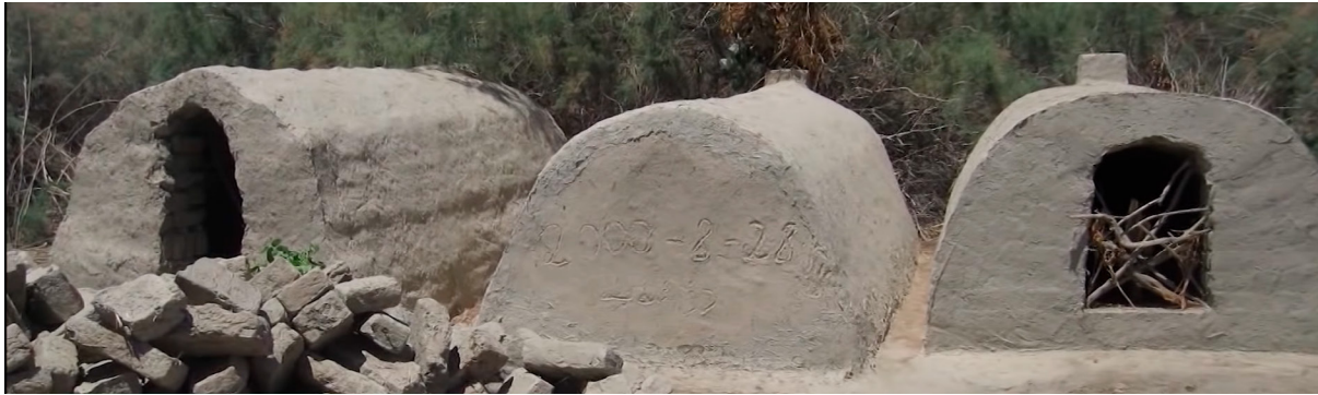
Figure 24: Dr Isa Abdulla's gravesite, before its demolition
