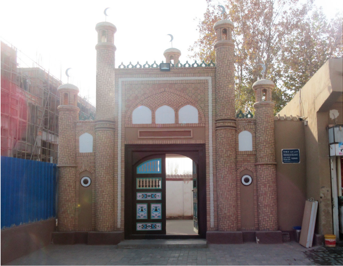
Figure 14: Kargilik’s Grand Mosque gatehouse rebuilt at a smaller scale in 2019
