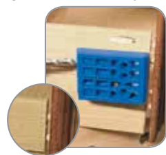
Drill pocket holes at the problem joint.
