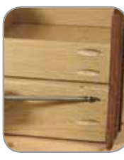
Drive self-tapping screws to secure the joint.
