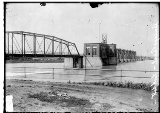
Near view of a bridge and locks on the drainage canal at Lockport, Illinois. This image was taken as part of a Chicago Railways Company Trolley Trip in 1908. Cite as: DN-0006895, Chicago Daily News negatives collection, Chicago Historical Society.
