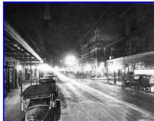
Night time on 7th Avenue in Ybor City, Fla. ca. 1927. Shown are automobiles in front of Henry Clay Shoe (1602 East 7th Avenue) and Smith and Smith Chiropractic. Also included are the street railroad tracks in the 1920s brick paving. A black and white photograph in jpeg format contributed by: Burgert Brothers. System number B29-unk-00000021
