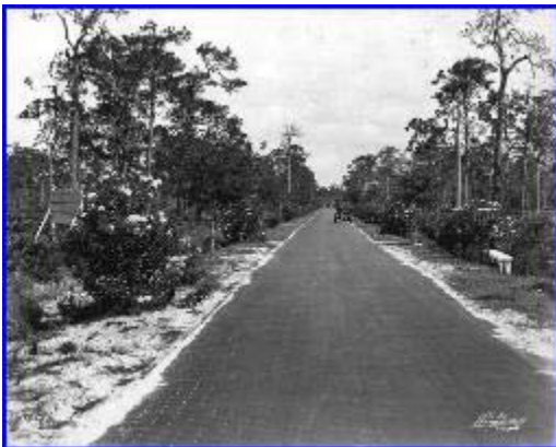
Brick paved Memorial Highway built on sand through a forest grove. Photo taken ca. 1920s. A black and white photograph in jpeg format contributed by: Burgert Brothers.
