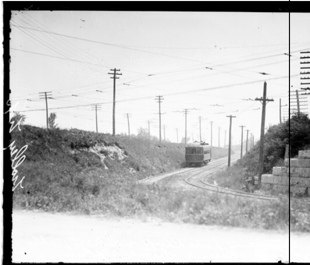
View of a trolley driving on the Milwaukee and Racine electric road between Lake Bluff and Libertyville, Illinois in 1908. This image shows the trolley driving through a rural landscape with many electrical wires overhead. This image was taken as part of a Chicago Railways Company Trolley Trip. Cite as: DN-0006821, Chicago Daily News negatives collection, Chicago Historical Society.
