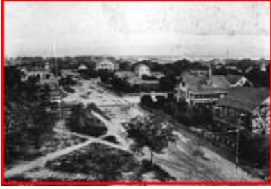
An Aerial view of a dirt street (later Hyde Park Avenue) passing through a residential area of Hillsborough Bay, Fla. Houses have already begun appearing in this area at this time of the picture. A black-and-white photo in jpeg format in the Burgert Brothers Photograph Collection. Unique Identifier: B29-rel-00000217
