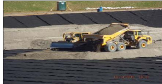
Placing Protective Cover
