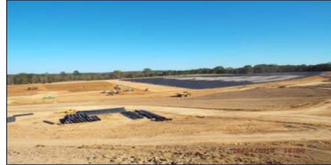
50% of Liner installed
