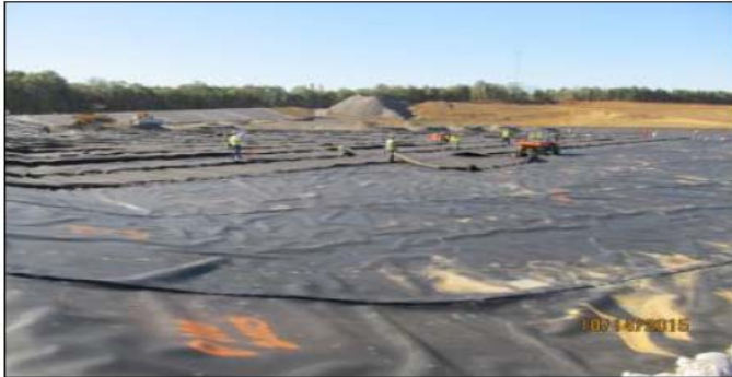
Installation of Geocomposite
