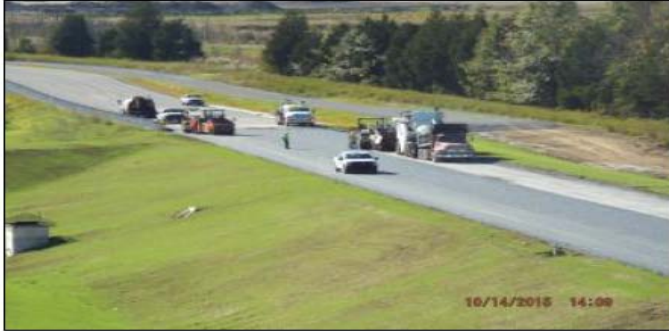
Haul Road paving
