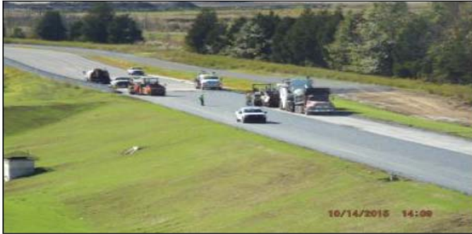
Haul Road paving
