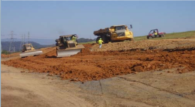
Construction of Improvements at Bull Run
