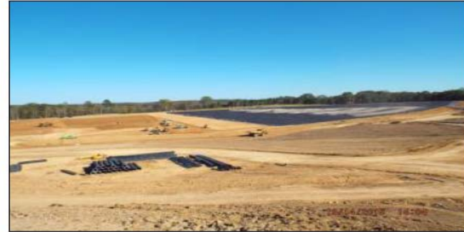
50% of Liner installed
