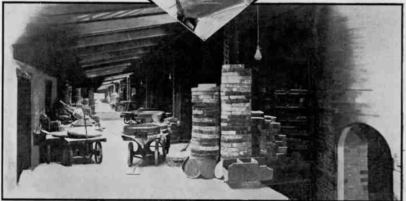
A row of great vitrifying kilns in which the abrasive wheels are placed. The kilns are brought to the required temperature by a coal fire which is placed underneath them
