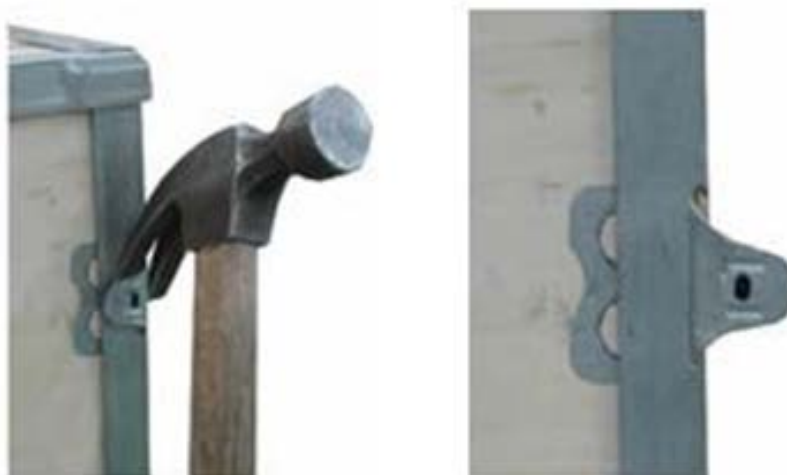
Figure 2-7 Straightening the hook
