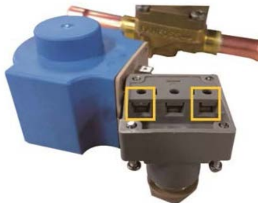
Figure 2-23 Connecting the cables of the Solenoid valve
