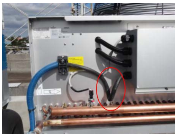
Figure 2-36 Condenser Wiring
