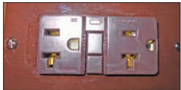
Figure 9-13: GFCI receptacle
