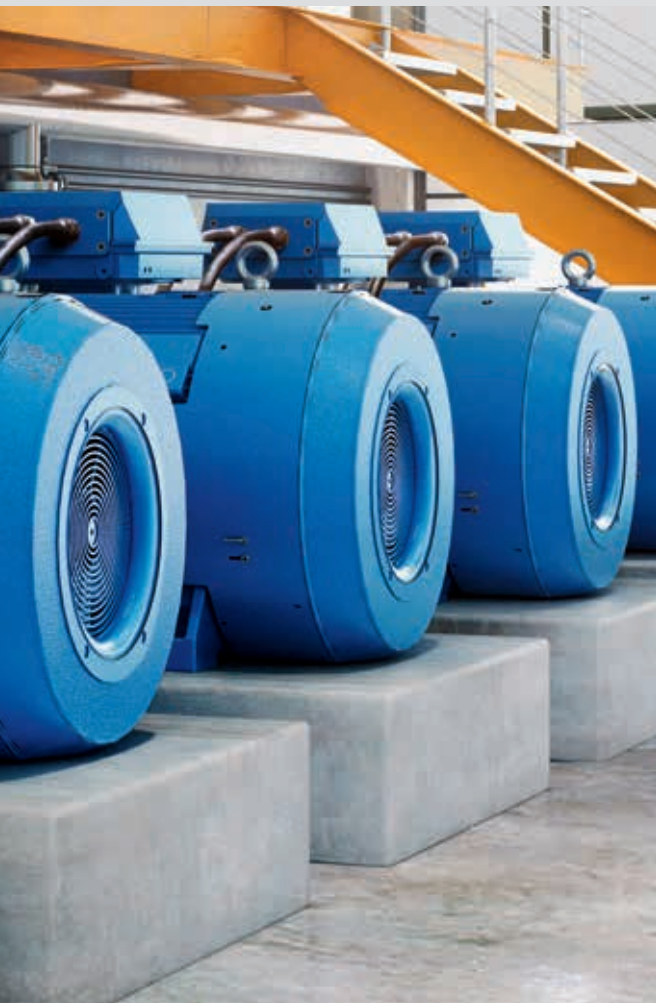
— 03 Smart sensors monitor the health of low voltage motors.
