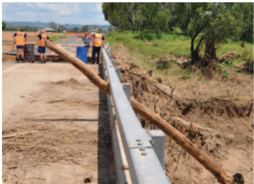
Image: John Parkin asks a local across the broken Kapernick's Bridge if he still had service following the Grantham Flood - he did.
