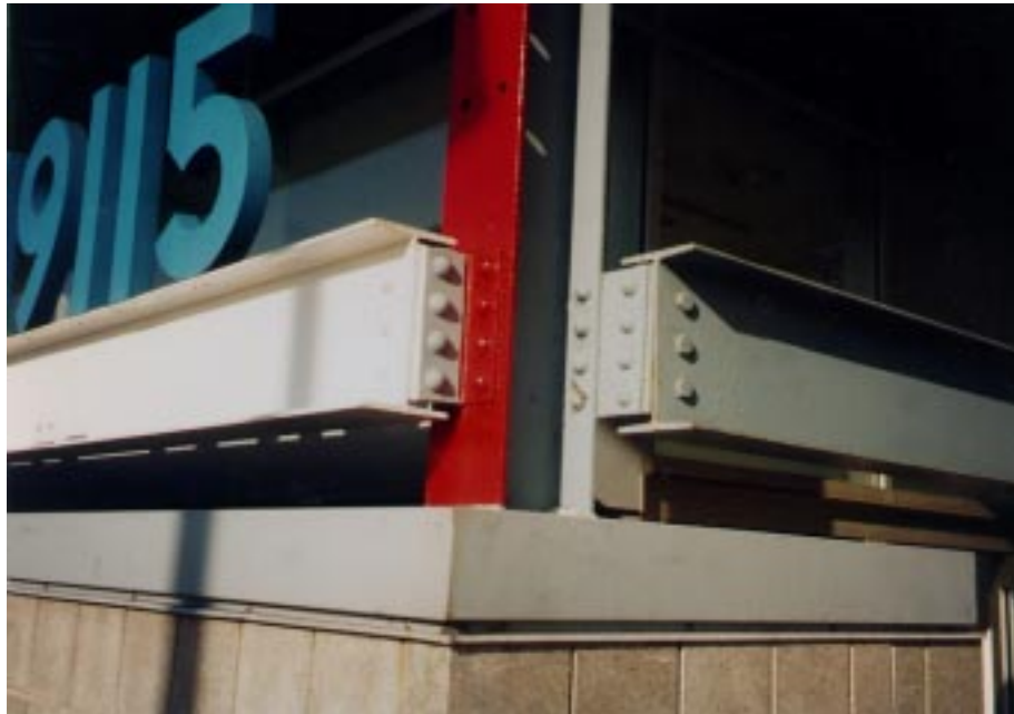
Exhibit 5 Building Construction - Detail Shot
