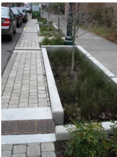
Examples of stormwater devices integrated with street design.
