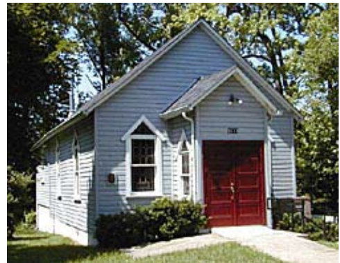
Ridgley Methodist Episcopal Church Source: Prince George's County Historic Preservation Program
