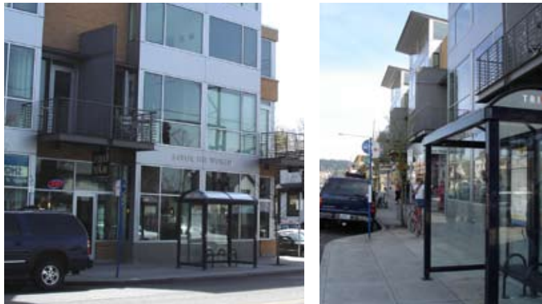
Bus Stop Improvement Examples
