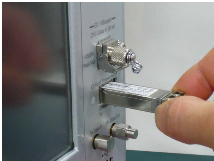
Figure 2.8.1-1 Installing Optical Transceiver
