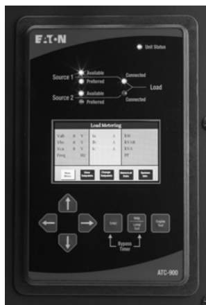
ATC-900 Main Screen Shows Current Values
